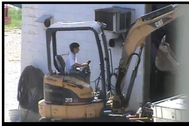
A 10-year old boy operating heaving machinery in Florence, AL.
