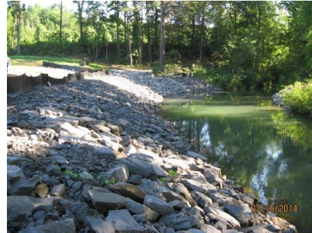
View east of the southern portion of the project site with Blue Creek returned to its original stream bed after reclamation of the Adger Slope Portal Emergency.
