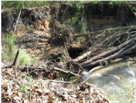
View northwest of the reopened Adger Slope Mine Portal with Blue Creek flowing into the opening. Note eroded and sloughing banks of the stream associated with flood water activity.
